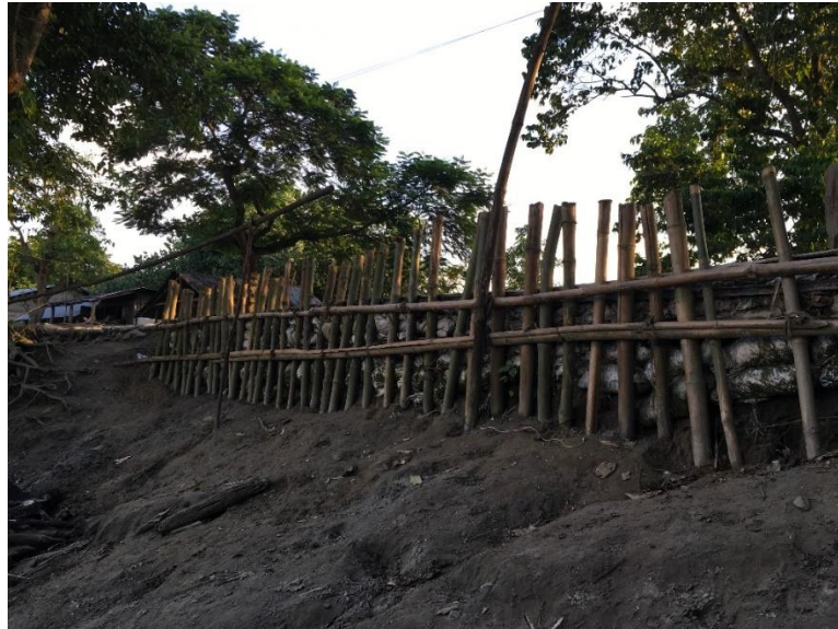
Community effort to stabilize the embankment in Majuli
