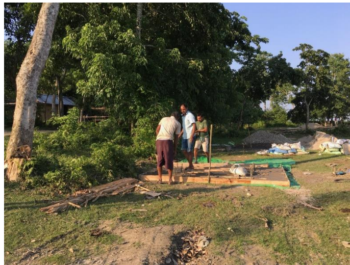
MGNREGA work of strengthening embankments done by men
