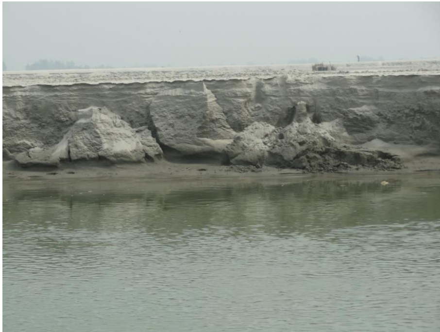
River erosion in the Char causing frequent and extensive losses of land
